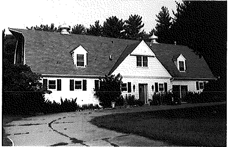
16. Residence (renovated barn)
