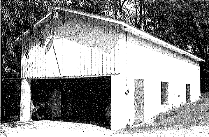
2. Garage (adjacent to Brady Lodge)
